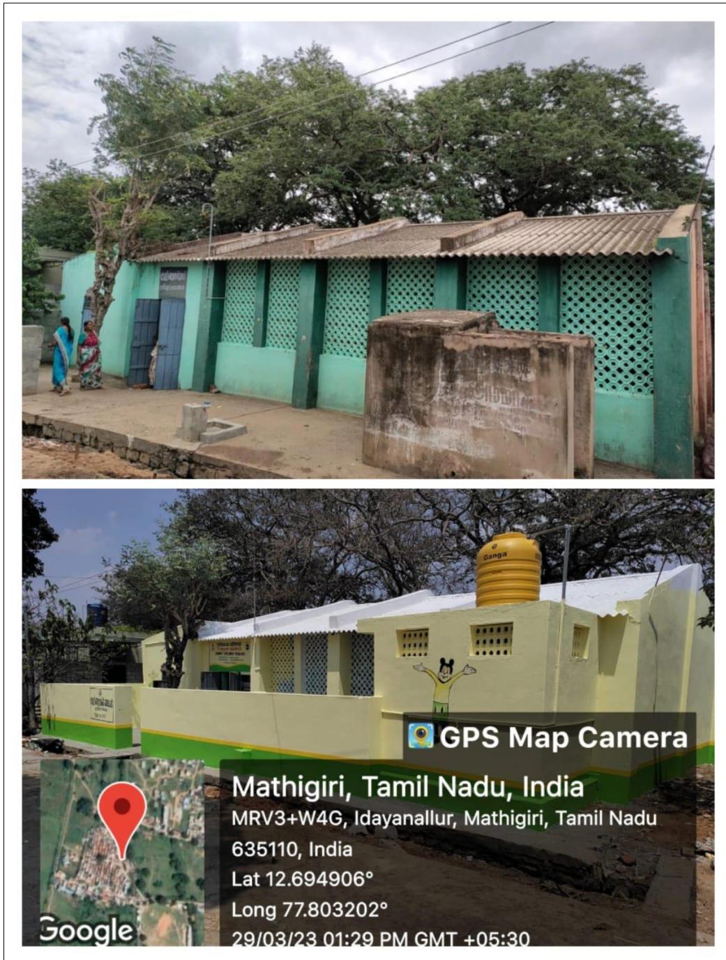
A renovated Anganwadi building at Kudirepalayam village
